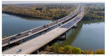
Circle Drive Bridge consisted of rehabilitation of both east and westbound spans of the bridge deck and barriers and repairs to the deck soffit while managing the busy demands of summer traffic.
